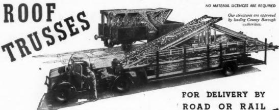
S.M.D. have specialised in the production of  $22\frac{1}{2}^{\circ}$  pitch aluminium alloy roof trusses. This has enabled continuous production of trusses with spans up to 60 feet to be maintained, with the result that delivery times of eight to ten weeks from receipt of order can now be offered. The largest order in production is for 650 identical trusses.
