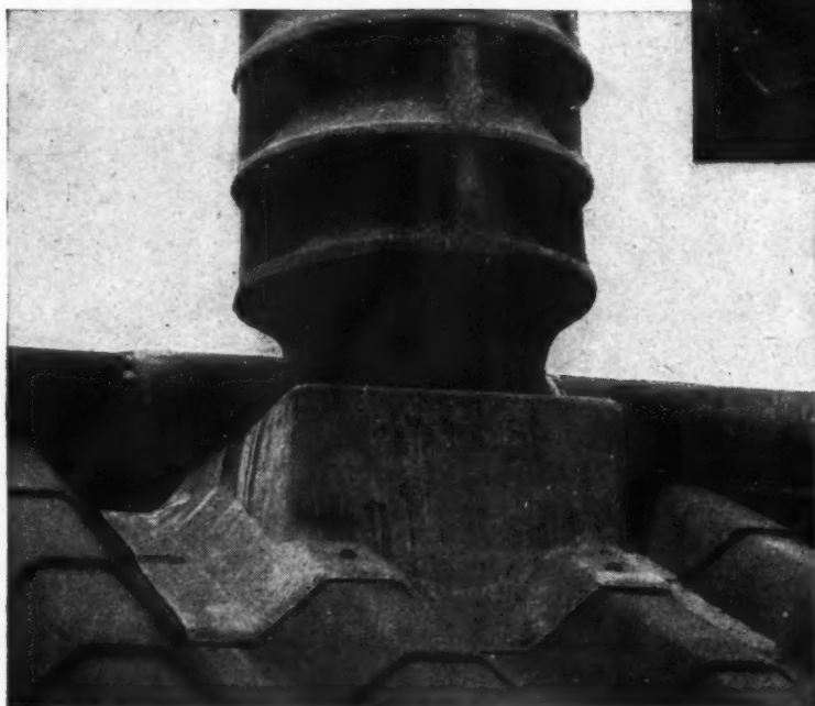
Two recent and widely differing examples of chimney flashings in sheet lead.
