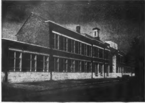
Boys' High School, Rock Ferry, served by Leonard-Thermostatic Water Mixing Valves.
