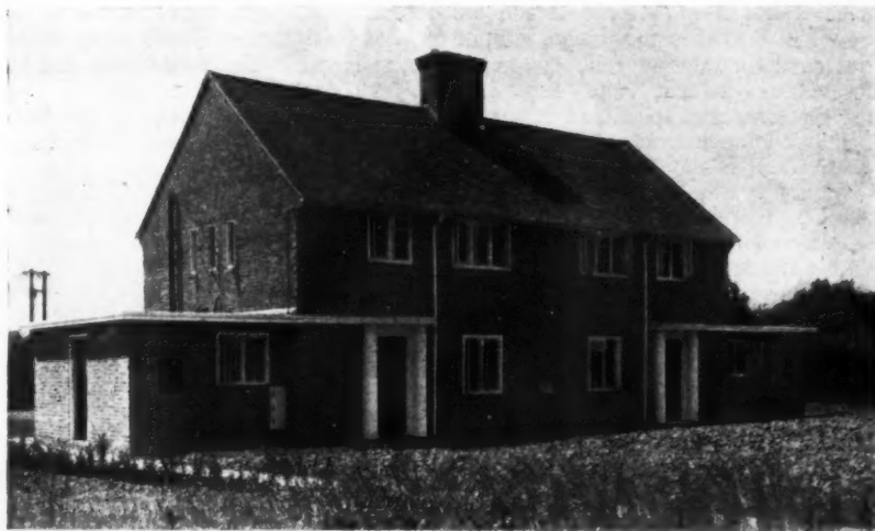
Demonstration houses at the Close, Ardingly, Sussex, built by E. H. Munmin, Ltd.; designed by L. Keir Hett, F.R.I.B.A., and planned specially for rural areas in Southern England. They are built of bricks made in the district.
