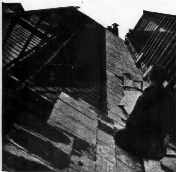
Two views of the roof of a weaving shed. The contract was in Lancashire for approximately 1,500 sq. yds. of roofing consisting of eleven bays each approximately 190 ft. long.
