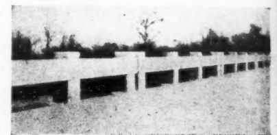
Bridge Railings in the USA. Top, the curb furnishes adequate protection to vehicles, and height of railing gives protection without spoiling the view. Centre, smooth wall provides a good barrier and design allows wide scope in treatment of top rail. Below, for rural bridges a single wide rail projecting inside the posts provides protection and is economical. See No. 2593.
