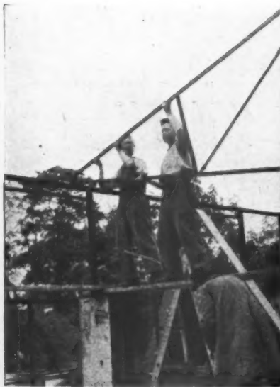
Left, placing a prefabricated roof truss in position. Centre, bolting the framework. Right, the interior cover strips of which a detail is shown on the following page.
