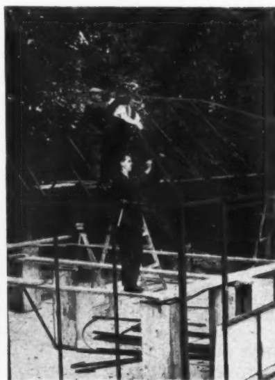
Left, placing a prefabricated roof truss in position. Centre, bolting the framework. Right, the interior cover strips of which a detail is shown on the following page.
