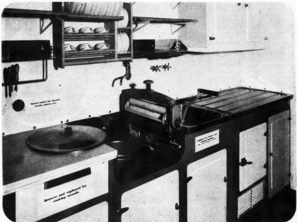
A close-up of the kitchen side showing clothes boiler, sink and wringer in position.
