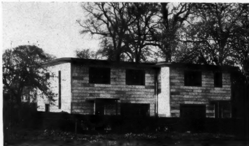
The Airey House will be shown in the Hall of Houses at the Modern Homes Exhibition to be opened at Dorland Hall on March 26. The house embodies a system of frame construction with a cladding of pre-cast vibrated reinforced concrete panels and is one of four permanent prefabricated houses to be shown in the exhibition in the form of models. The Airey House is by Richard Costain Ltd. The exhibition is being organised by the Daily Herald.
