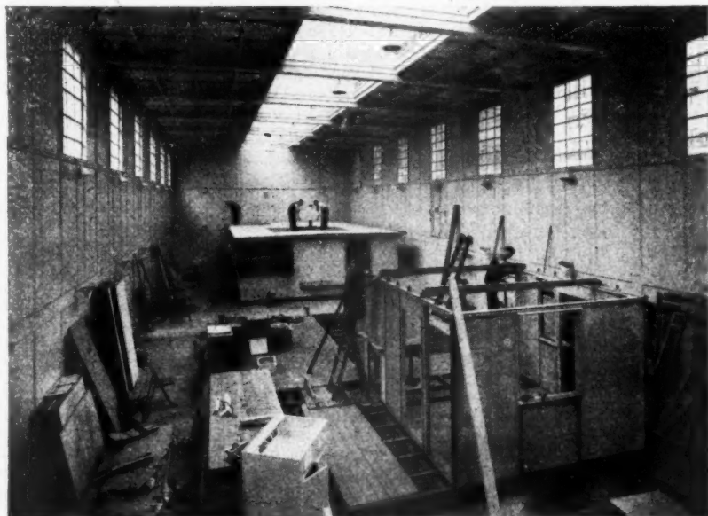
The Uni-Seco Training Centre in Park Lane. Regular courses are held on the Uni-Seco methods of construction. The photograph shows prototypes of the houses, which are erected for demonstration purposes.
