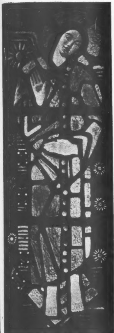
A new type of Aureole Window of thick pieces of stained glass set in reinforced concrete. See No. 2278.
