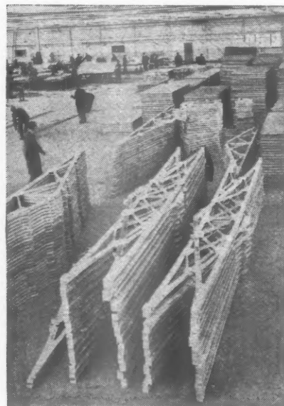
An inspection bay: roof trusses and wall panels awaiting final check.
