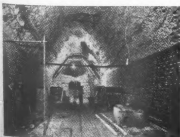
Constructing an underground factory in a tunnelled chalk hillside. See News Item.
