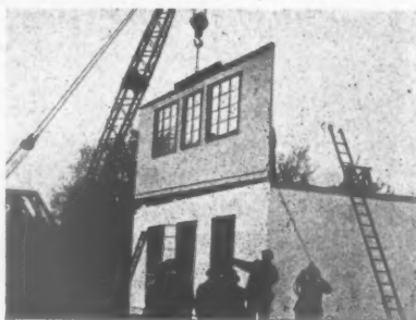
Left, erection of the Scottwood Plywood House at 9 a.m. on the second day, when the first floor and roof are completed. Below, two detail sections showing the joints at first floor and roof levels. See No. 2182.
