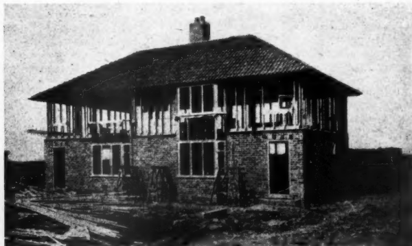
Two progress photographs in the erection of the Dennis steel-framed houses. Left, the steel framing, with its twin-trussed beams in the roof, carrying all super-imposed loads. Right, timber or aluminium studs in place with 4½ in. brick infilling up to first floor level. The internal skin is of 2½ in. foamed slag forming a 2½ in. cavity. See No. 2090.
