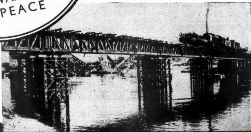
Bridge near Canello, on the Rome- Naples main line. Length 400ft.
