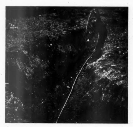
Installation costs of domestic water supply services will be much reduced by the use of "KUTERLON" Long Length Copper Tube which is now supplied in coil form in lengths up to 60 ft. Annealing for the use of mechanical bending appliances are not necessary. Bending can be done by hand,
