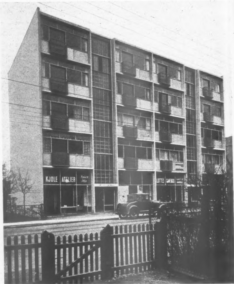
Top left, diagram of Box Frame construction applied to flats. Above and left, flat buildings in Copenhagen built before the war on the Box Frame principle. Top, Architect: Mogens Lassen, Structural Engineer: Ernst Ishoj. Left, Architect: Hubert Paulsen, Structural Engineer: Ernst Ishoj.
