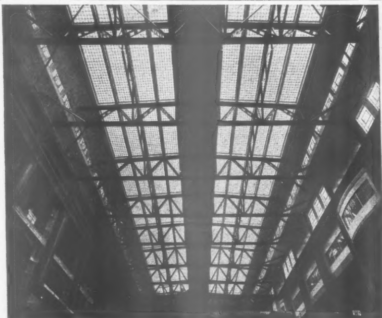
The illustration is of the roof to the turbine house at Fulham Power Station where many thousands of sq. ft. of GLAS-CRETE constructions were installed. The construction shown is double glazed in order to minimise the risk of condensation which is a vital point in connection with electrical machinery.
