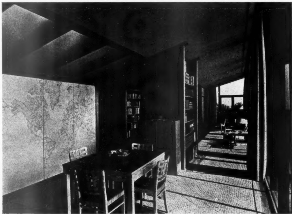
Top, the living room illuminated by the laylight which provides diffused fluorescent light at night and sunlight in the morning ; ceiling covering is asbestos cement sheeting of natural colour ; walls are covered with redwood both inside and out. Below, looking across the dining room into the living room ; there is a buffet behind the map-covered doors and behind that again a wide hatch to the kitchen ; there is a built-in loud-speaker above the cabinet.
