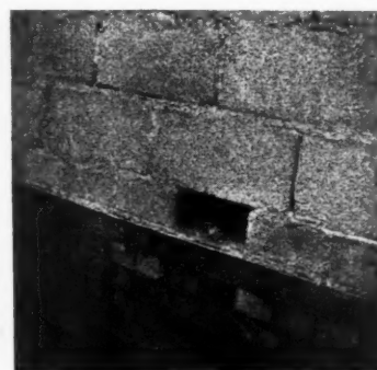
Above left, buttering a block with cement, lime and foamed slag mortar. Above centre, a chimney stack during construction showing parged flue. Above right, the plinth below the DPC of ordinary brickwork ; above the DPC is a course of foamed slag briquettes forming a continuous hollow which collects any moisture within the walls ; this escapes through open joints ; during construction a few briquettes are left out, so that the hollow can be cleared of droppings. Below left, a view of the finished job. Below right, a gable end during construction.
