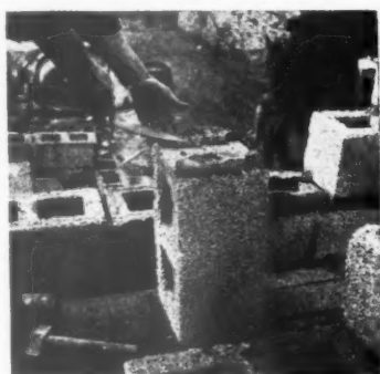
Above left, buttering a block with cement, lime and foamed slag mortar. Above centre, a chimney stack during construction showing parged flue. Above right, the plinth below the DPC of ordinary brickwork ; above the DPC is a course of foamed slag briquettes forming a continuous hollow which collects any moisture within the walls ; this escapes through open joints ; during construction a few briquettes are left out, so that the hollow can be cleared of droppings. Below left, a view of the finished job. Below right, a gable end during construction.
