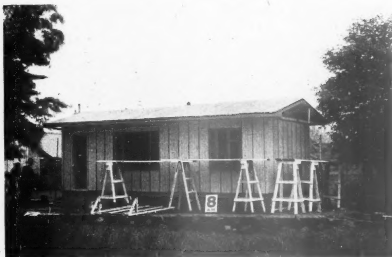
This experimental bungalow was erected complete with fittings in Hull in one hour. It contains living-room, two bedrooms, kitchenette and bathroom, and is built of the Tarran system, which was described in the A. J. for July 27. Top, all parts assembled on the site at 7 a.m. Left, the building is up by 8 a.m. Below, the completed house.
