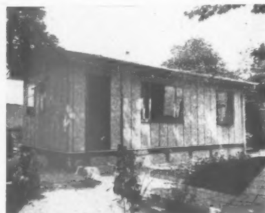
This experimental bungalow was erected complete with fittings in Hull in one hour. It contains living-room, two bedrooms, kitchenette and bathroom, and is built of the Tarran system, which was described in the A. J. for July 27. Top, all parts assembled on the site at 7 a.m. Left, the building is up by 8 a.m. Below, the completed house.
