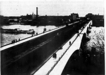
Waterloo Bridge now open to six lines of traffic, its full width, as compared with three lines on the old bridge. The building of the new bridge was begun in October, 1937, and has continued despite the difficulties caused by war conditions. But for the war the bridge would probably have been completed in 1940. The present parapet railings are temporary.
