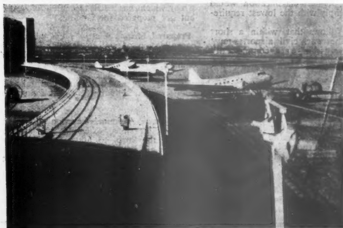
An elevated walkway at the terminal building of La Guardia Field, New York.
