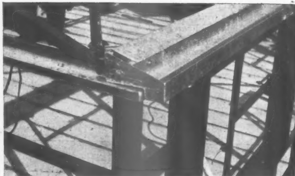
Left above, detail of steel foundation frame. Before concreting, the frame is levelled by means of screw-jacks which are integral with the steelwork. The shanks of the jacks can be seen projecting. Right above, detail of zinc gable flashing and eaves flashing. The gutter is integral with the flashing.
