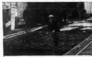
Economical of labour—one man can lay and interlock the sheets.
