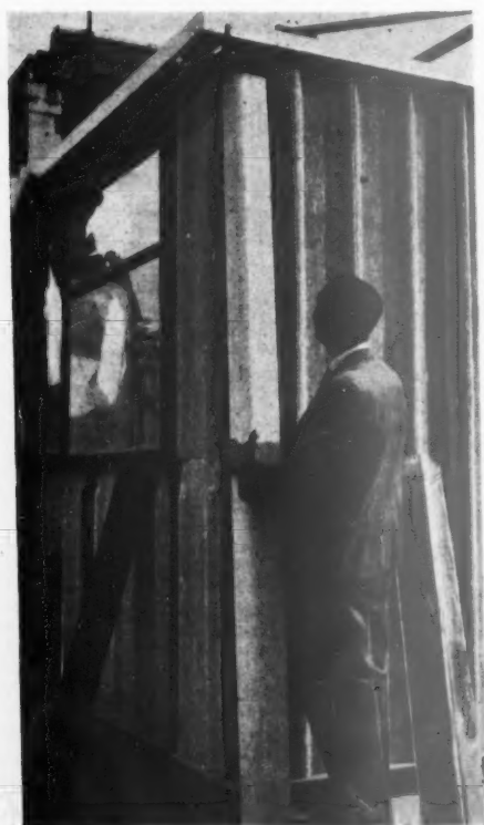
Above, general view of the main entrance front. The canopies over the doors are of painted asbestos cement. On the left of the main entrance is a unit of steel framework, extending from floor to eaves; the panels, which are not glazed, are of insulated sheet steel. Below, a view during construction, showing the angle unit and the inner asbestos cement skin.
