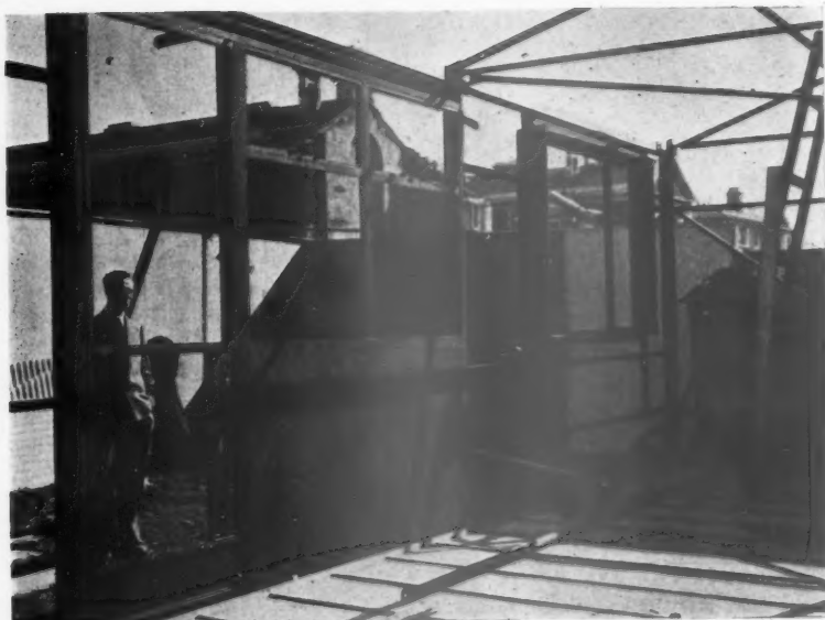
The steel framework during erection. The steel windows and surrounds are made as part of the framework. A steel unit forms the outside wall of the bathroom and w.c.
