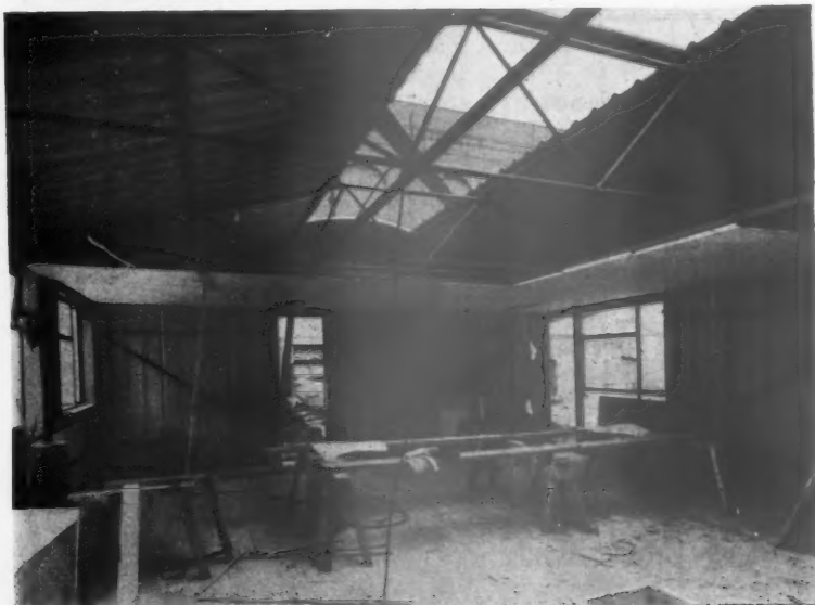
Interior view during erection. The ceiling panels are being fitted into position, being suspended from the trusses by a system of main and secondary T-section steel bearers which makes for quick erection.
