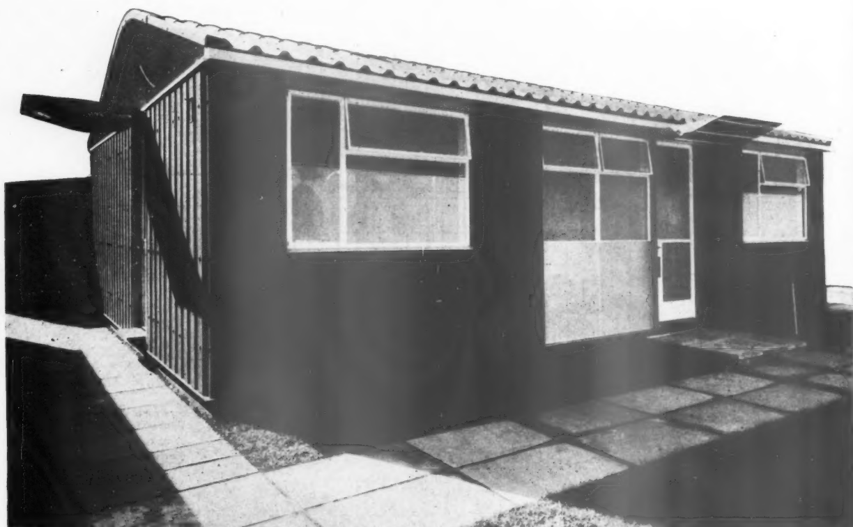
Above, general view of the main entrance front. The canopies over the doors are of painted asbestos cement. On the left of the main entrance is a unit of steel framework, extending from floor to eaves; the panels, which are not glazed, are of insulated sheet steel. Below, a view during construction, showing the angle unit and the inner asbestos cement skin.
