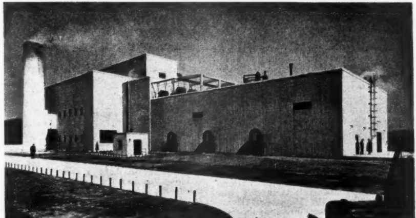
The second power plant at Wright Aeronautical plant at Lockland, Ohio. The shortened stack is made possible by induced draft fans. Architects: Albert Kahn, Architects and Engineers Inc. See No. 1670
