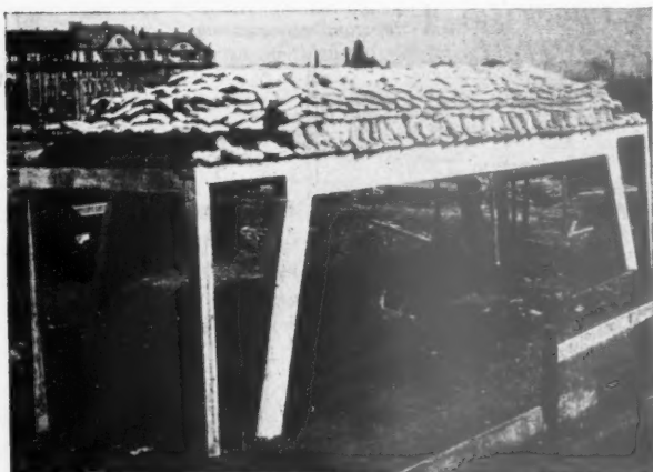
8 Preliminary test model of the Market Hall, Frankfurt, to a 1:3 scale.
