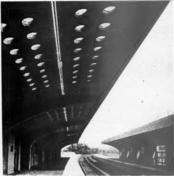
19 Malden Manor Station, on the Southern Railway, is an example of a cantilevered roof in shell construction.
