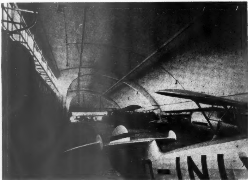
14 An aircraft hangar in Germany with an asymmetrical arch.
