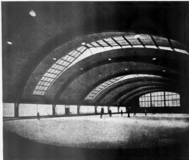
25 The ice-rink at Haverford, Pennsylvania, of shell roof construction with glazing.
