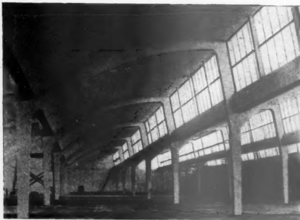
22 A later extension of the factory shown in Figs. 20 and 21. The spacing of the columns was doubled here and the window area reduced by 25 per cent.
