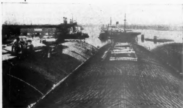
12 A shell roof in Hamburg under construction, showing the reinforcing rods of one of the barrel vaults.
