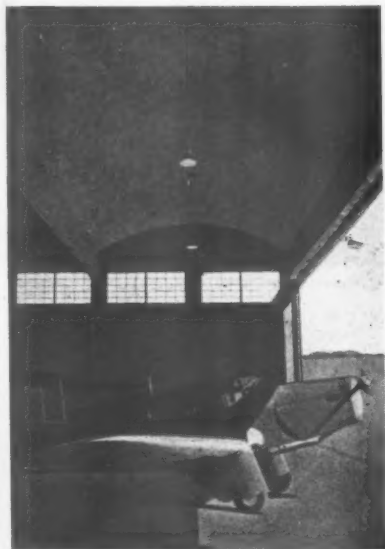
15 An aircraft hangar at Doncaster Municipal Airport. Each arch spans 30 ft. The length of the barrels is 90 ft. The thickness of the shell is 2\frac{1}{2} in., which encloses three layers of steel rods.
