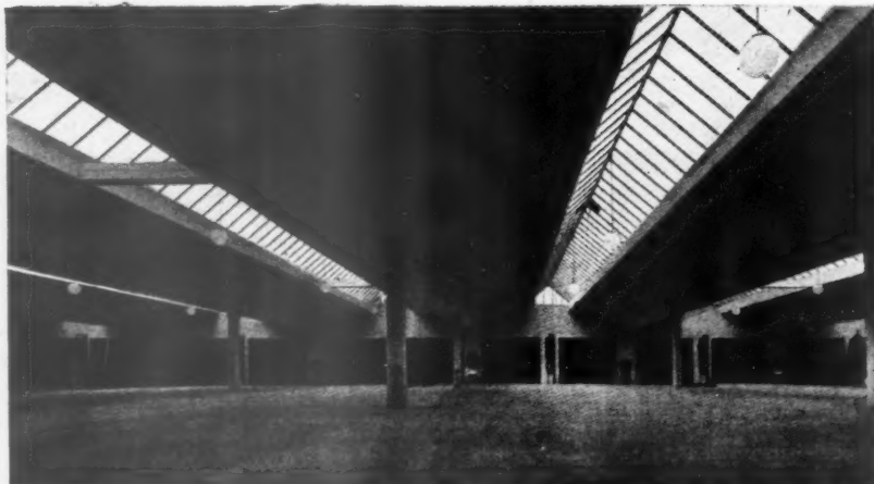
17 A bus garage at Nürnberg. One column carries a roof area of about 240 sq. yds. Pumice concrete was used here to improve the thermal insulation.
