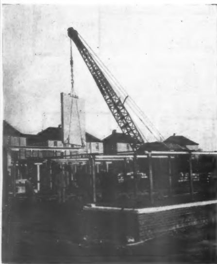
Top, front elevation of completed block. Above, a precast wall unit of reinforced foamed slag concrete being lifted by a crane for stacking, after being removed from its metal form.
