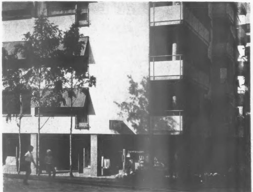
High densities involving flats in central urban areas are not necessarily undesirable provided advantage is taken of living close together to provide amenities and equipment not usually possible with houses. This is an example of eight storey flats in Stockholm.
