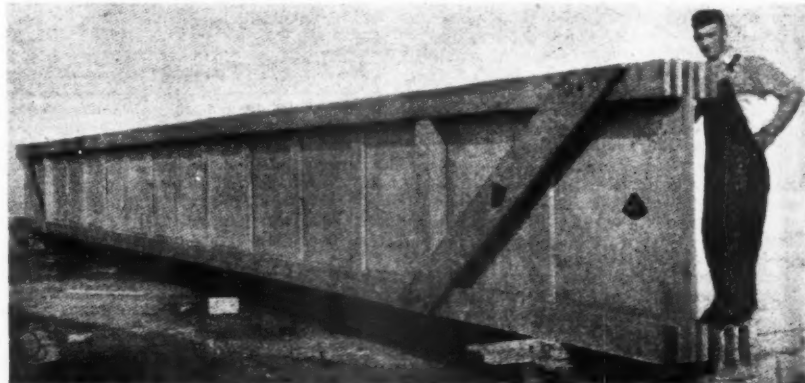
This USA plywood plate girder, 60 ft. long by 6 ft. high with a 1½ in. plywood web, carries a load of 1,200 lb. per lin. ft. See No. 1402.
