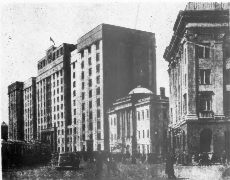
Fig. 1. The general height of buildings on the Sadovoya ring-road is being increased with a result that some of the smaller buildings are dwarfed in scale. If the buildings are of architectural or historic interest, they are to be moved to new sites as, for instance, in the case of the building in the centre, next to the new offices of the People's Commissariats.
