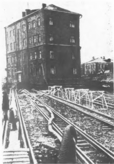
Fig. 10. No. 12 Great Pioneer Street being moved. The flexible rubber connection maintains the drainage system during the move.
