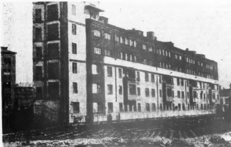
Fig. 4. A block of flats moved in 1937 to make way for the new approach to Kvarnholm Bridge. The building was moved 144 feet through an angle of 19°. The curved railway tracks on which it was moved can be seen in the foreground.
