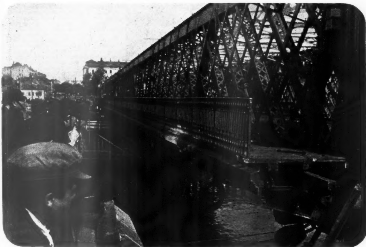
Above, the removal of the Krinsky (Crimean) Bridge, Moscow, to a new location in 1936. This bridge of welded iron, built for horse traffic, has been replaced by a new steel bridge. In order to avoid a traffic hold-up, the old bridge was moved some fifty yards down stream, while construction of the new bridge was going on. The photo shows the moment when the bridge, having been raised about 9 in. and mounted on steel supports, was moved 10 yards on the first stage of its journey.
