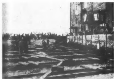
Fig. 6. A building at the Kim factory in Moscow moved in 23 days inclusive of preparatory works. A crowd of spectators watch in the distance.
