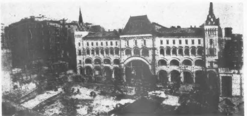
Fig. 21. The move completed with the railway lines, on which the building has travelled, cleared away. The original position of the building is indicated by the hoarding in the left foreground.
