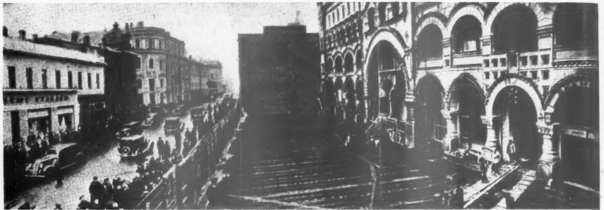
Fig. 20. No. 24 Gorky Street being moved back to allow road widening. The building is shown on the way to its new site.
