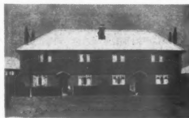
A block of four three-roomed Weir steel houses of the Blanefield type built at Lochend, Edinburgh, in 1926-1928. See No. 1380.
