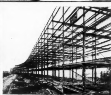
BOOTH STEELWORK FOR LEEDS MUNICIPAL FLATS
