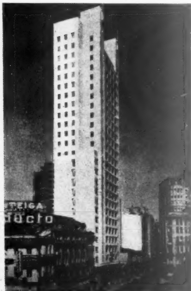
Serious settlement of a corner of this tall concrete building was recovered by jacking it on to new piers sunk through artificially frozen sand. (See No. 1375).
