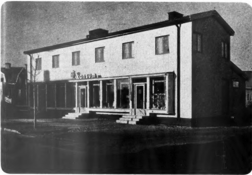
Left, a shop, with living accommodation over, made of prefabricated timber sections, in a Swedish provincial town. Below, sketch, ground floor and basement plans of a standard timber bungalow.
