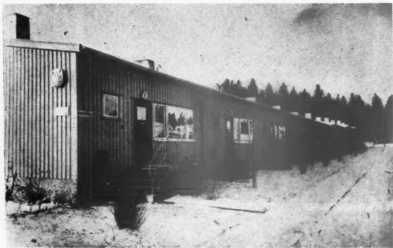
Terrace house types. Top left, family houses for the workers at Kvarnholmen, the Co-operative Society's industrial centre outside Stockholm. Top right, plan of one of these houses; 2, living room; 3, bedroom; 4, kitchen and dining alcove; 5, bath and wash-room; 6, terrace. Though the sections of these houses are of timber and prefabricated, the exteriors of the walls are rendered. Above, a terrace of small houses. Here the exterior is of the typical vertical timber boarding. Below, a bachelor hotel built by the Co-op. at Gustavsberg. The restaurant with its different exterior treatment is at the near corner.
