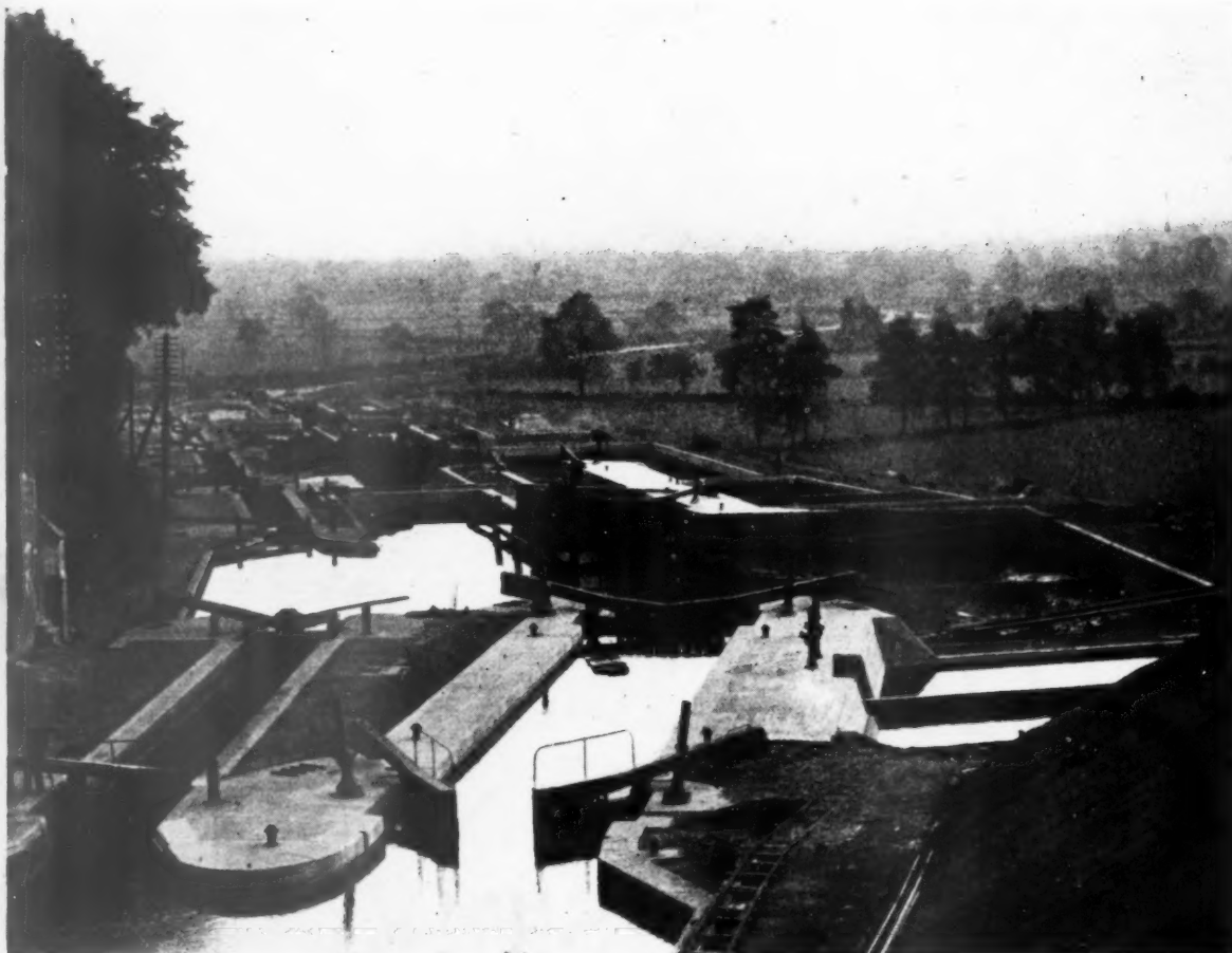
Reconstruction of canal lock in reinforced concrete.
