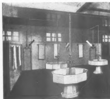
Leonard-Thermostatic hot and cold Water Mixing Valves serving ablution fountains.
