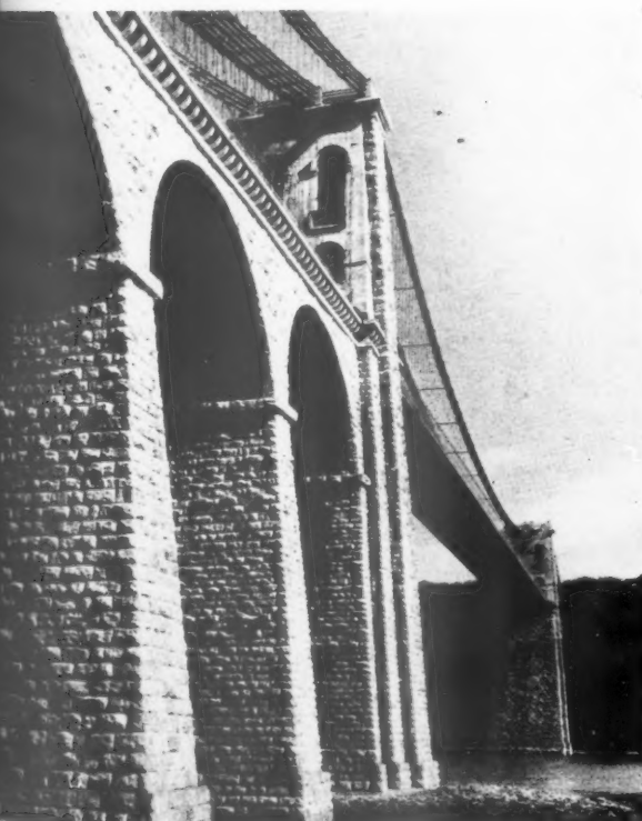
The first of the world's great bridges was completed in Britain in 1826. Telford's masterpiece, across the Menai Straits, has a span, between piers, of 570 feet.
