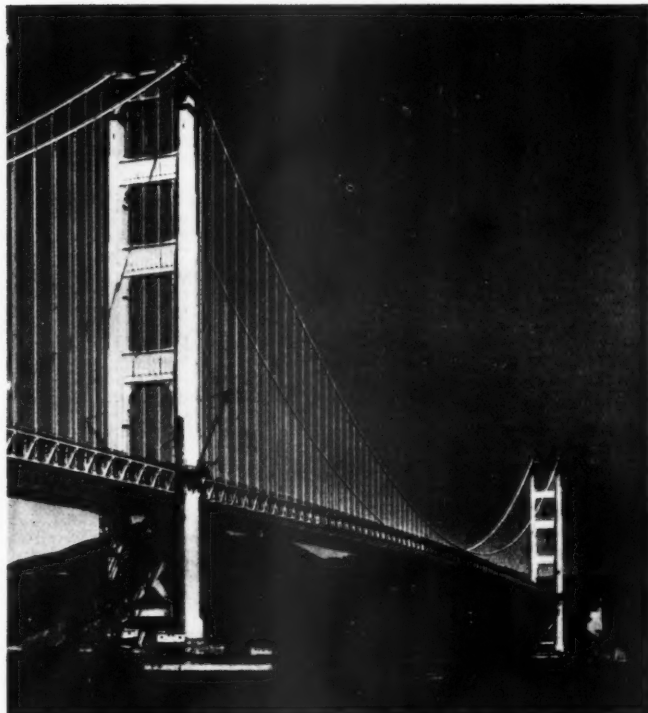
Golden Gate Bridge, San Francisco, U.S.A.—the world's largest suspension bridge. Twentieth century technique: clear span, four thousand two hundred feet ( \frac{1}{2} mile). Height of towers: seven hundred and forty-six feet.
