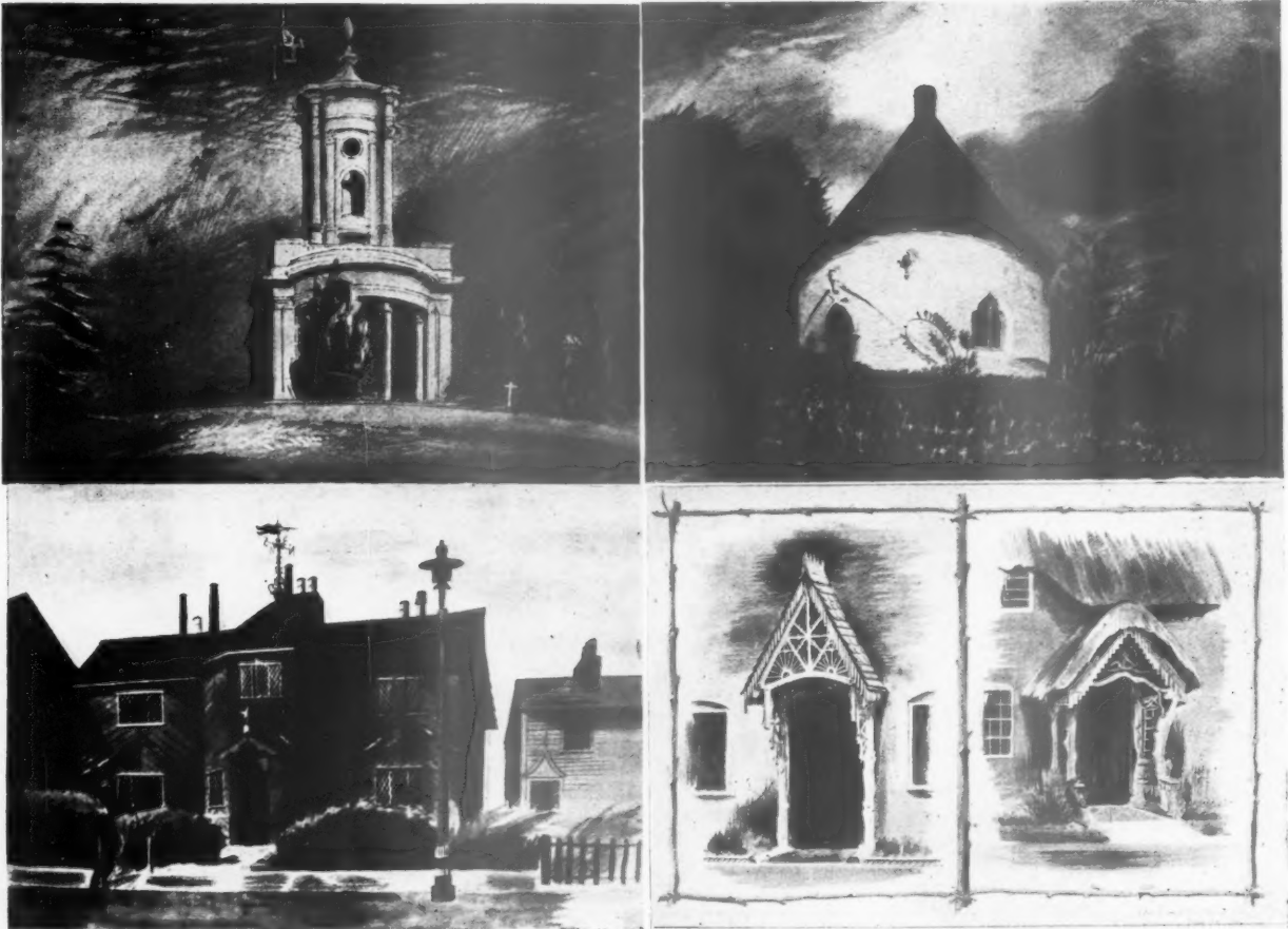
The third and final exhibition of selected drawings produced under the Scheme for a Record of Changing Britain is now at the National Gallery. Top left, church in the park at Normanton, Rutland, the western portico and tower of which were built in 1826; drawing by John Piper. Top right, the Round House, Veryan, Cornwall, one of the three Parson Trust's Houses; the present incumbent believes that they were built early in the nineteenth century by a lord of the manor who went to Africa and was impressed by the kraals; drawing by Barbara Jones. Above left, wooden houses at Carshalton dated 1758 by Barbara Jones. Above right, cottage porches at Canford Magna, Dorset; most of the cottages of this village have elaborate rustic porches, no two alike; drawing by Barbara Jones.
