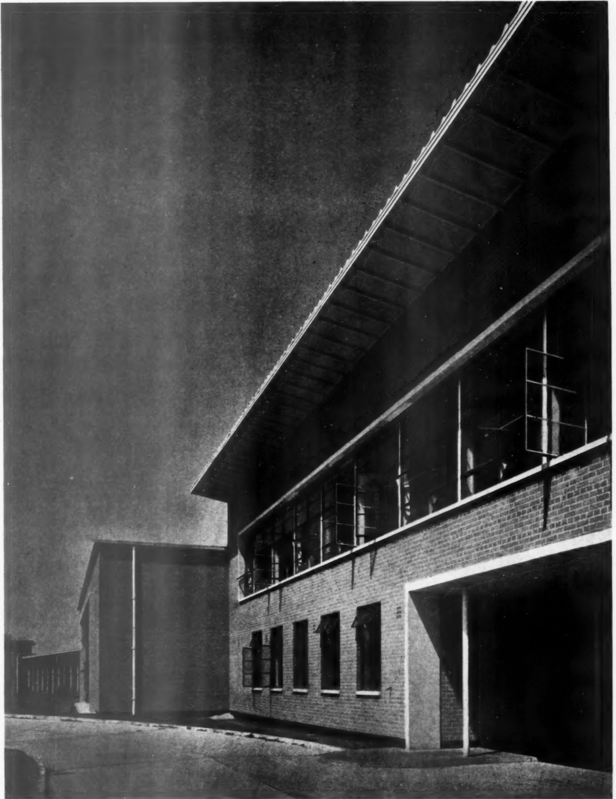
Above, looking along the principal front, showing main entrance through administrative block, to the left of which are the junior assembly hall and classrooms. Walls are faced with buff coloured cement bricks, classroom wings are light steel framed construction.
