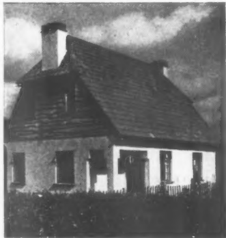
This cottage at East Bergholt provides a good example of the use of concrete in combination with other materials. Architect: H. R. Wheeler.
