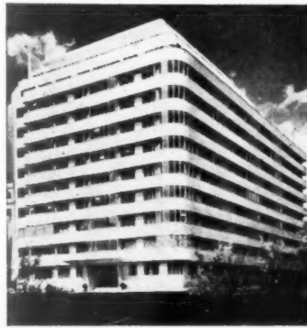
Embassy Court, Brighton. Reinforced concrete flats. Twelve storeys in height. The exterior of the building is faced with a light cream water-proof rendering. Architect: Wells Coates.
