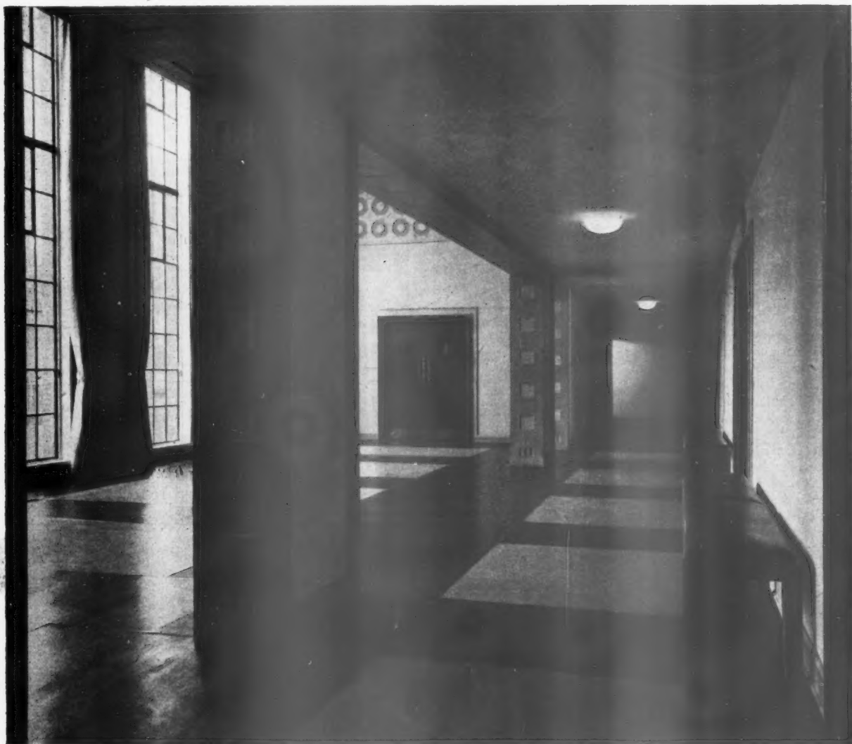
Above and facing page : two views in the entrance hall. The walls are finished with rough texture plaster, distempered beige colour ; the buff-coloured ceiling has rectangular panels inset with a geometrical design, decorated in light pastel shades of grey, green and slate blue. Floor is covered with black composition relieved by panels of the same material in beige.
