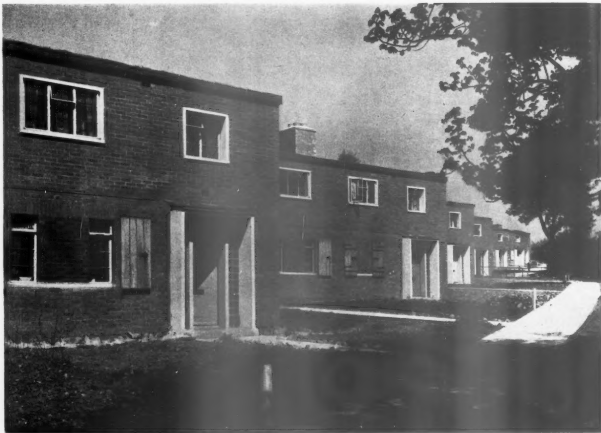
Semi-detached blocks. The staggered treatment affords better aspect and greater privacy. On facing page: Porch detail, showing the rendered finish which is the most usual throughout the site. On some other sites the wing walls have been carried out in facing brickwork or in white brick.
