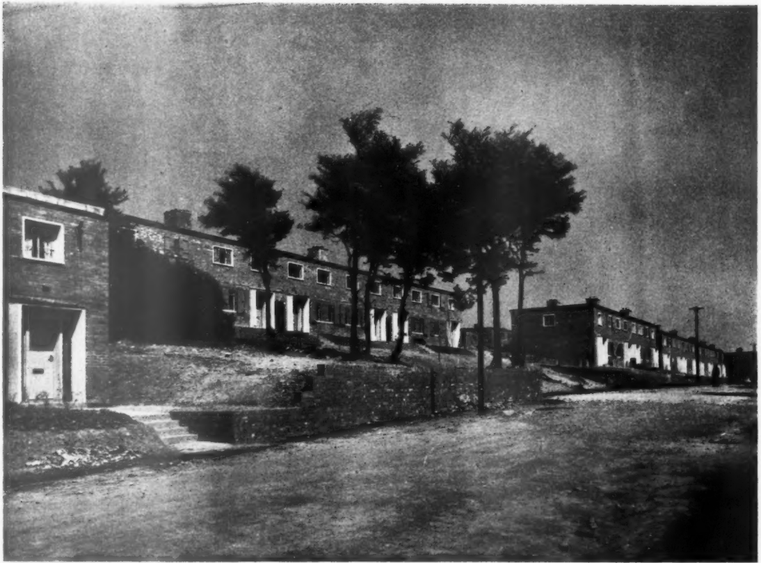
The long terrace blocks. The passages to the backs of the houses lie between the pairs of porches. The view reproduced below shows the treatment of a semi-detached block. The A.R.P. shutters will, of course, be removed after the war.
