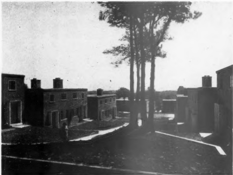
This view shows the sharply sloping site. The flat roofs allow the tenants of the upper houses a view of the landscape which would not have been possible if pitched roofs had been used. Below, the adaptation of the semi-detached block to a hilly portion of the site.
