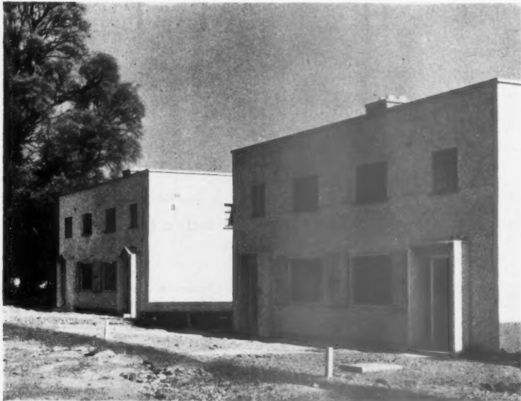
A variation of the standard design in Scheme 1, by Mr. T. Alwyn Lloyd, on a portion of the site for which he was consultant. The rendered finish and the extra weight of parapet above the first floor windows are the main variations.
