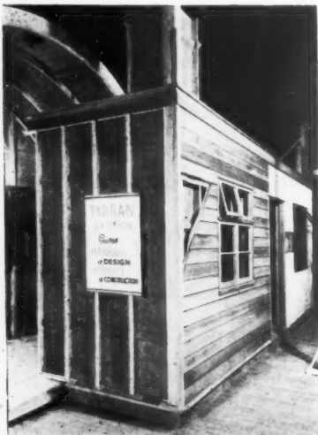
SECTION SHOWING INTERNAL AND EXTERNAL USE OF PREFABRICATED PANELS.
