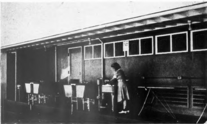
6 Provision is made for tenants to do their washing in the open-air. Here is a tenant using the wringer on the verandah of the washing block. Poles have been erected for the drying of clothes.
