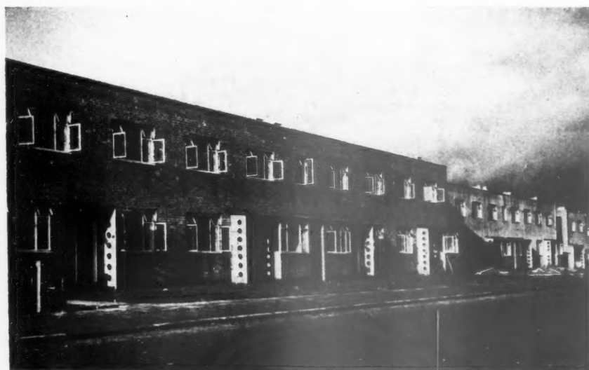
Above, two views of the preliminary scheme and a general view of the main elevation. Facing page, left, one of the precast concrete stair units used throughout the scheme: the lugs are built-in (note blocks let in for stair carpet holders), and column at back door; clay pipes are used as permanent shuttering. Right, view of porch showing space for perambulator.
