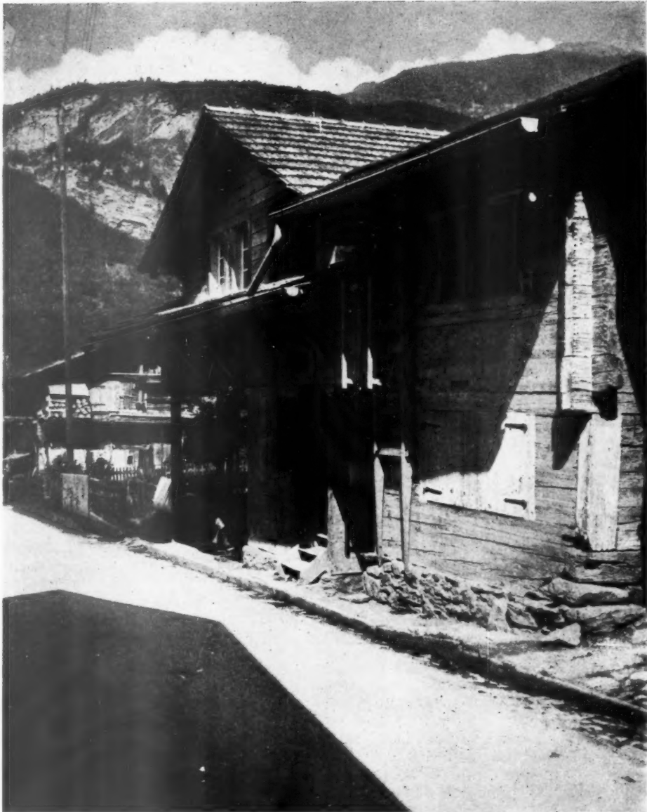
A chalet in heavy timber construction, most of the timbers being 8 ins. square, halved at the corners. The ground floor is used for stabling and storage with living accommodation over.
