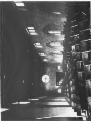
Nave looking west
