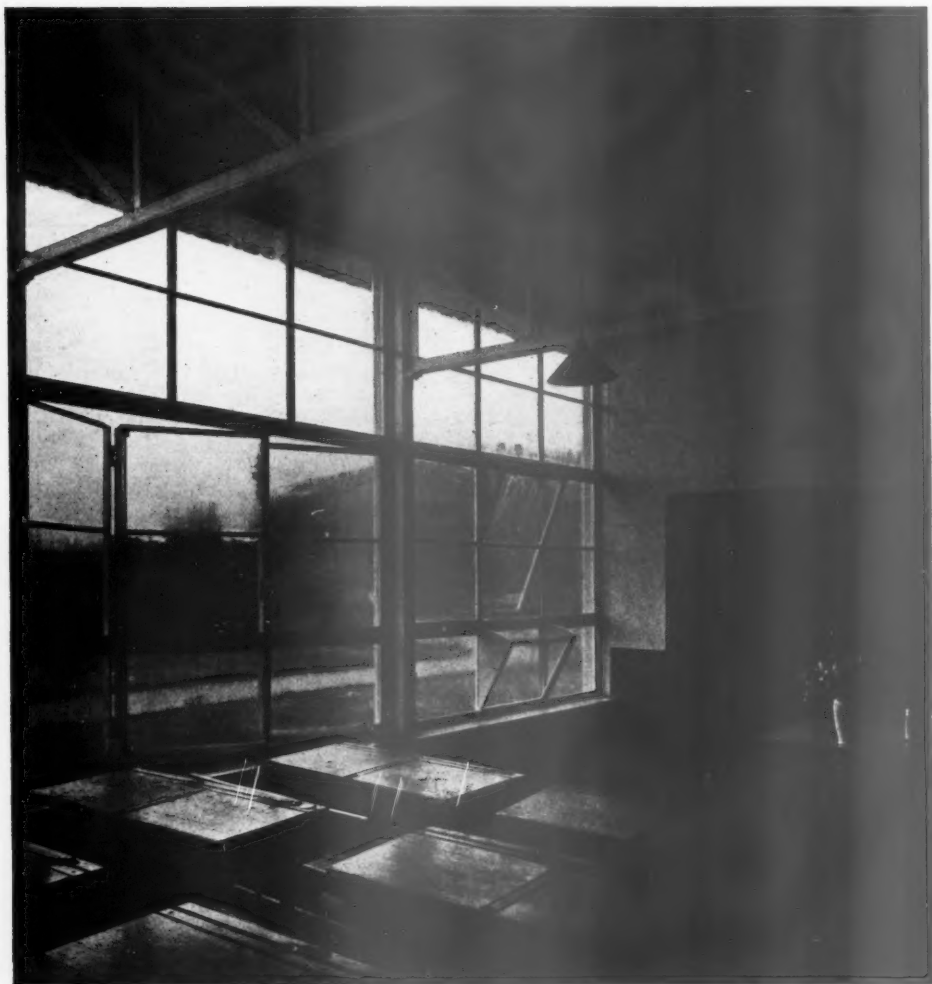
Left, a typical classroom. Below, left, the assembly hall looking towards the stage; right, a typical cloakroom.
