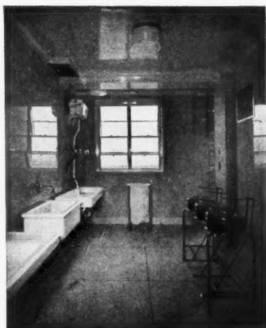
floor finished with cream terrazzo. 7: Typical sluice room; finishes—cream eggshell tiling on walls, with enamelled walls above; floor, quarry tiles. 8: Wash-up next to the operating theatre; vitrolite wall linings (green) and terrazzo floor (cream).
