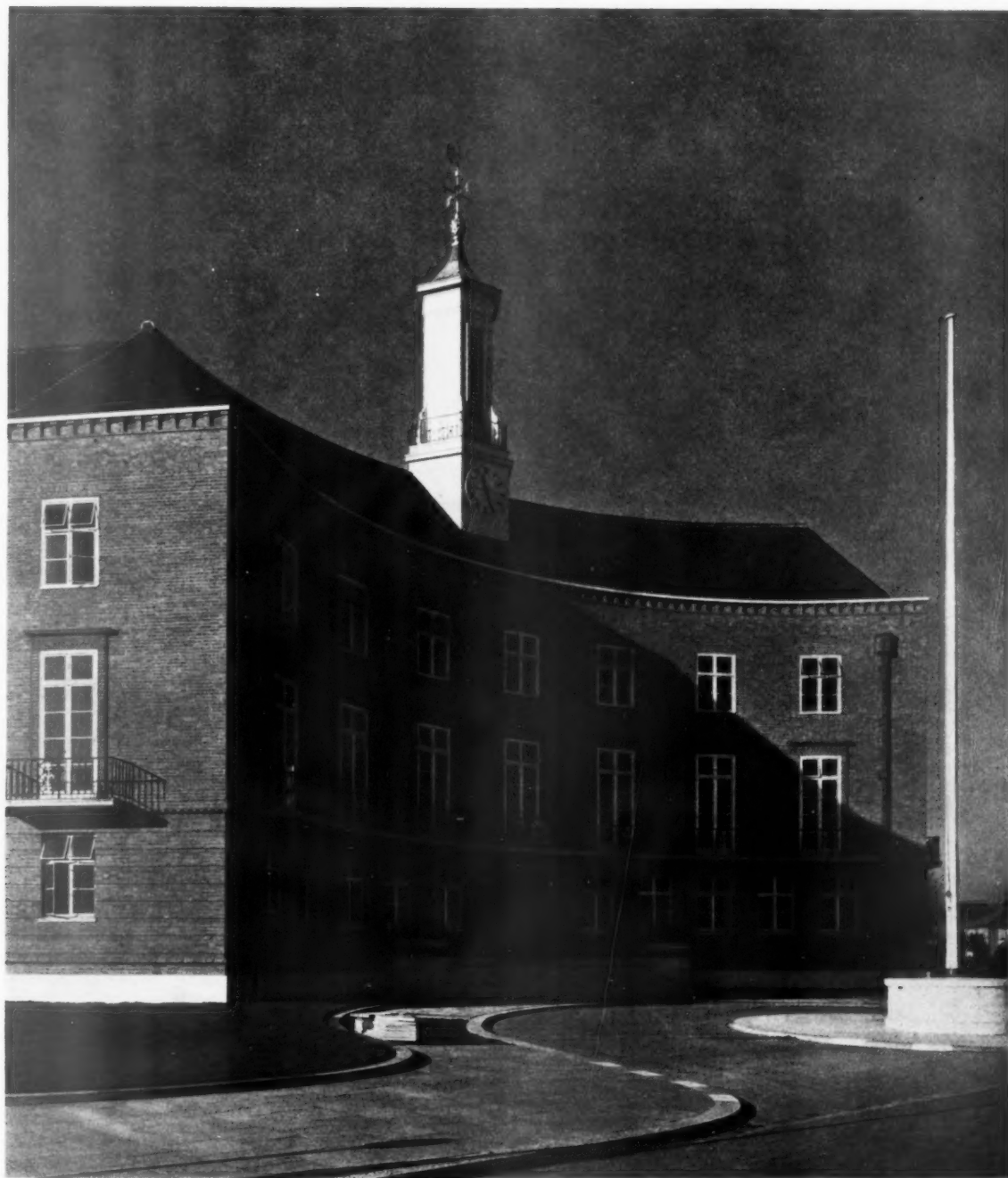
Main entrance to office block
