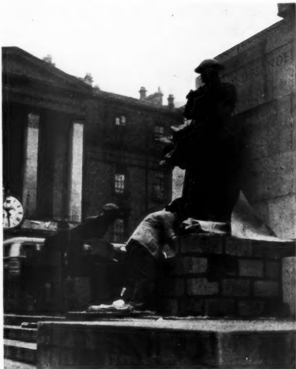
Concrete hollow blocks being erected to protect the Royal Artillery Memorial at Hyde Park Corner.
