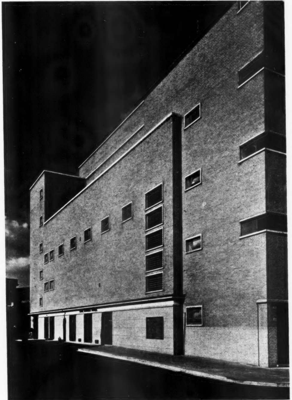
ABOVE : SOUTH FRONT. LEFT : VIEWS FROM THE SOUTH-EAST (TOP) AND NORTH-WEST.
