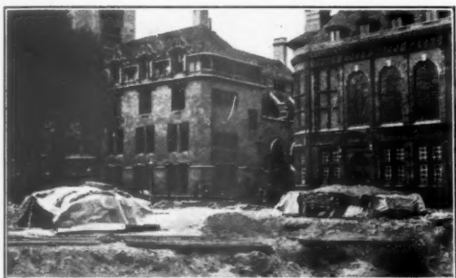
Protecting stocks of sandbags with Sisalkraft.
