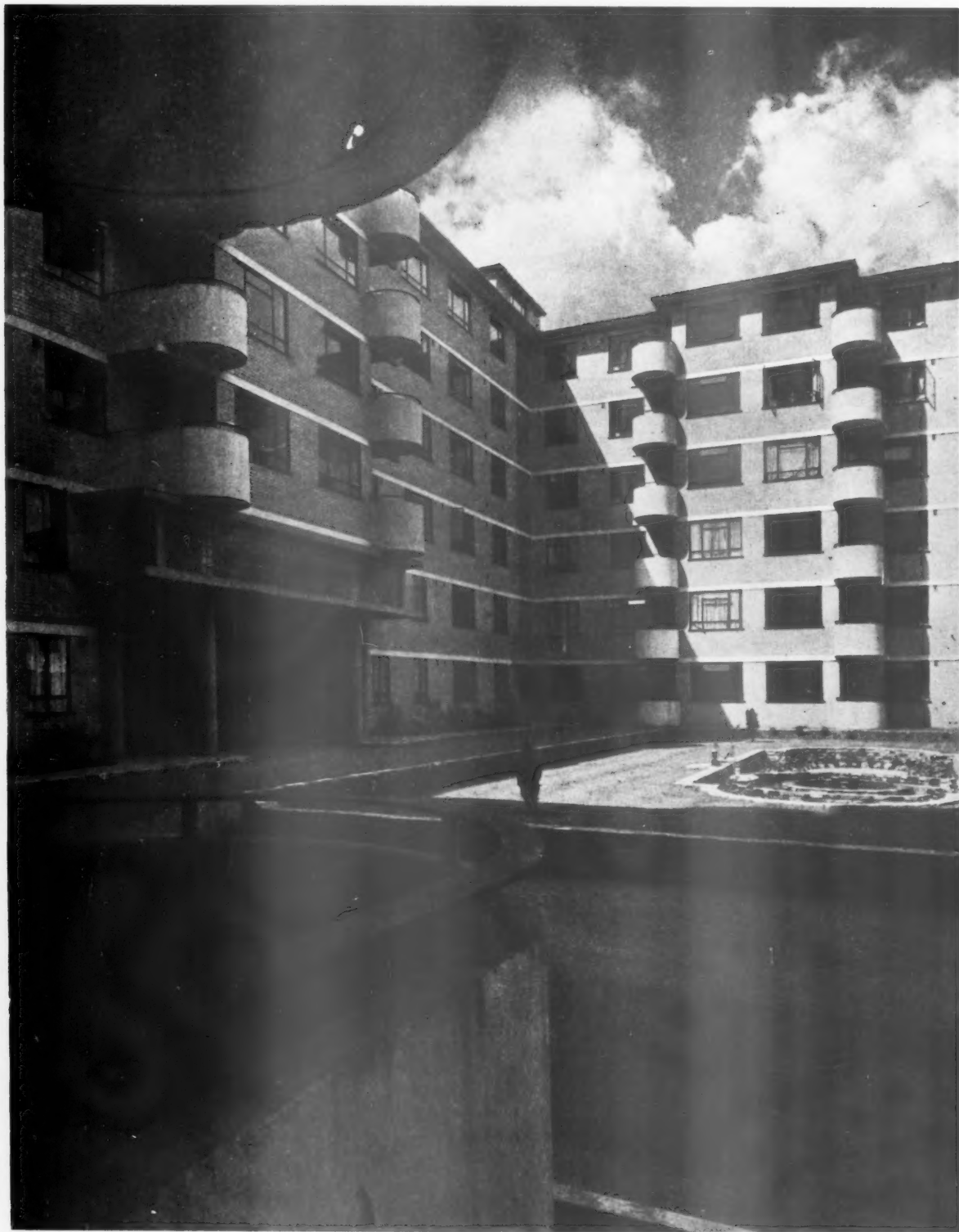
VIEW IN INTERNAL COURTYARD SHOWING ENTRANCE FROM CHRISTCHURCH ROAD
