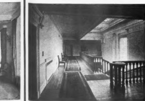
FIRST FLOOR LANDING
