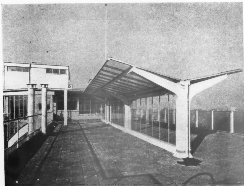
Open air treatment area on the roof of a Rotterdam clinic, by Brinkman and van den Broek. [From "Bouwkundig Weekblad Architectura."]
