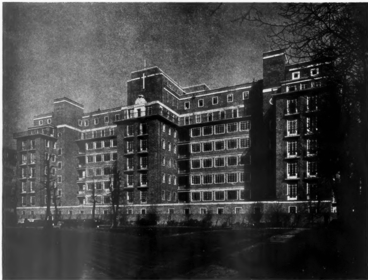
Elevation to St. John's Gardens.
