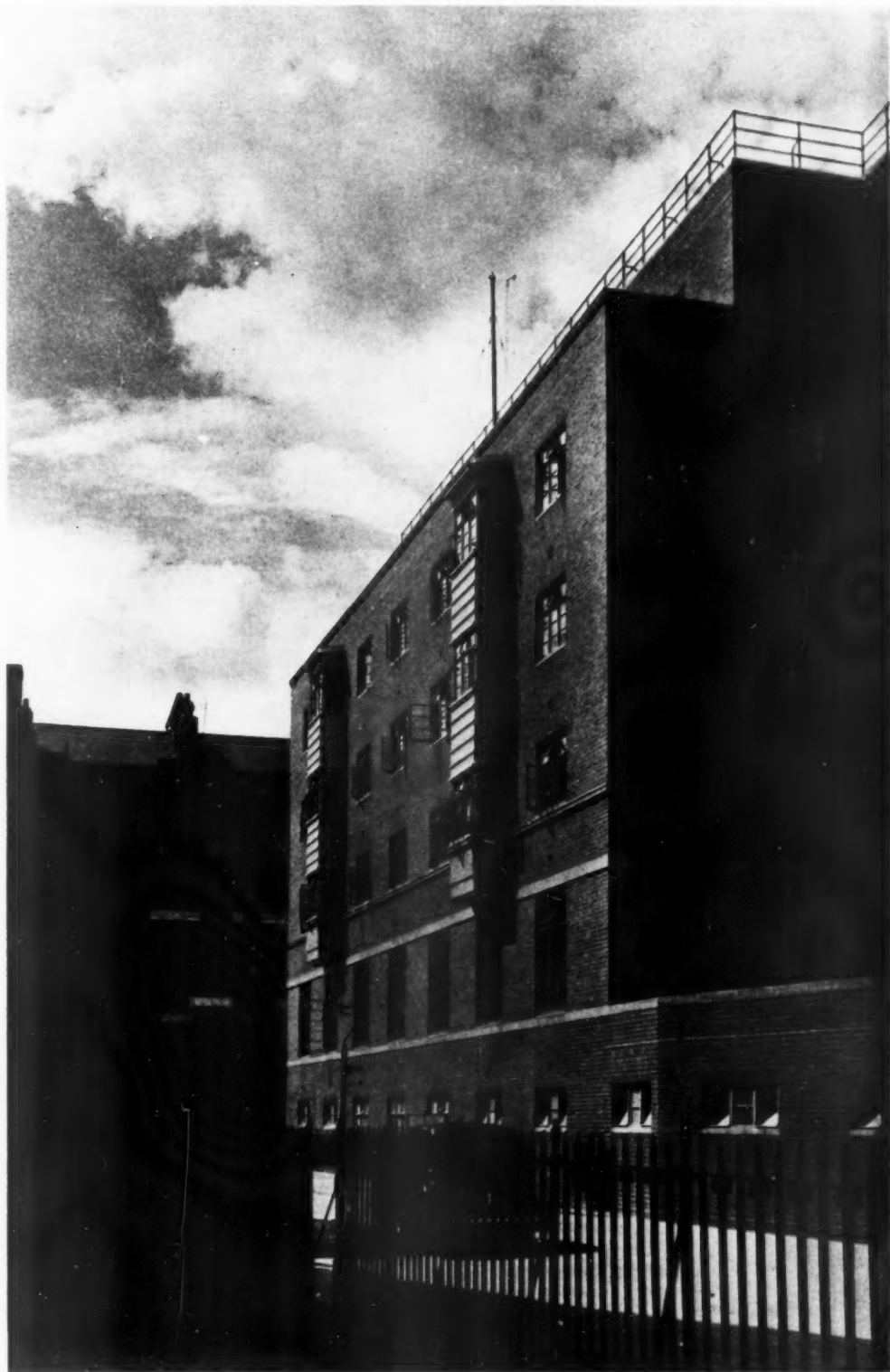
Part of the Compton Place front. Portland stone is used for the copings and strings. Brick and stone facings are tied back to the frame by dovetailed anchor slots and keys. Reconstructed stone is used for strings, copings and dressings on all elevations except this.
