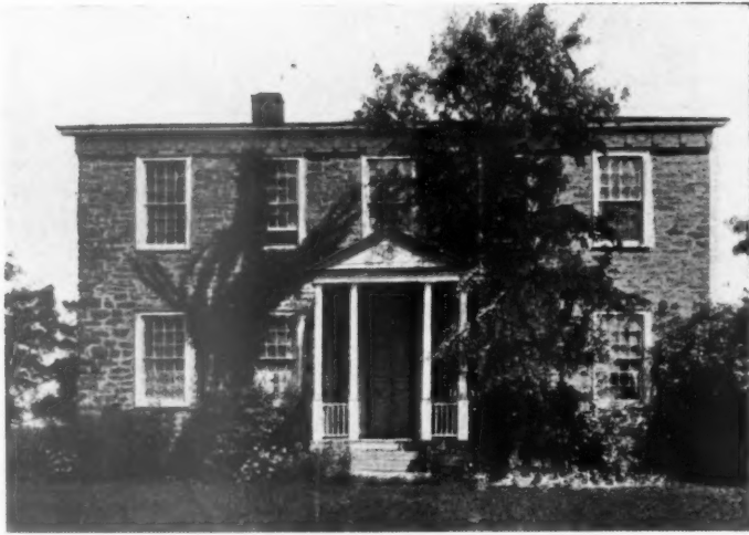
Poplar Hall, Maitland, Ontario. Early 19th century. Windows are on the outside face of walls with deep panelled reveals inside. Roof is slightly pitched: the porch is probably a later addition. From "The Early Buildings of Ontario."
