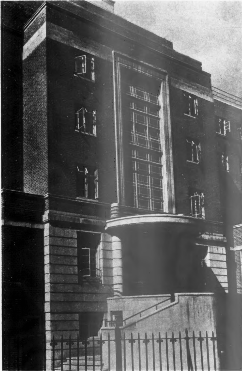
The recessed doorway to the main entrance from Compton Place has a reinforced concrete canopy. The stone balustrade to the entrance steps has bronze handrailing supported on turned and moulded balusters. The fanlight above the doorway has a decorative bronze grille.
