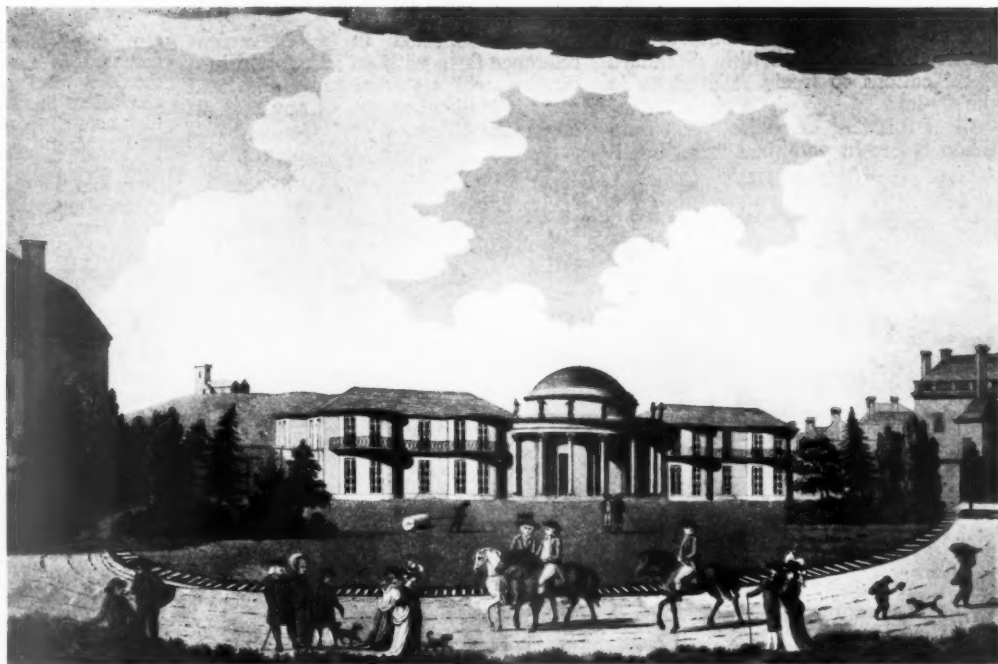
Royal Pavilion, Brighton: the east front as designed by Holland, showing the Castle Ball Room to the left and Grove House to the right. By Middleton, after Holland, 1788. Below, ground floor plan.
