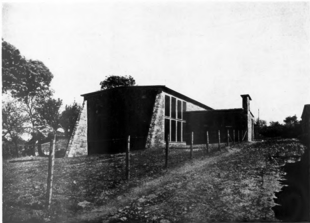
A chapel in Leversbach, by Rudolf Schwarz, built from local materials by the villagers themselves. (From the "Architectural Forum.")
